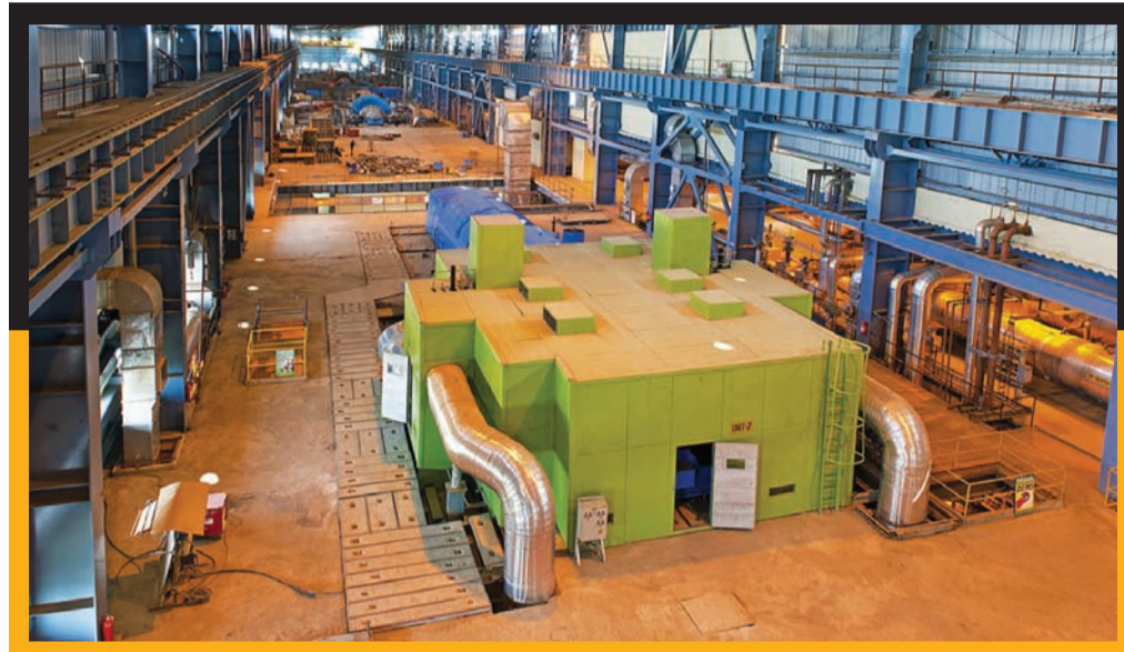
▲ An inside view of the Amravati coal-fired power plant whose phase-I comprising five units of 270 MW stands fully commissioned.
