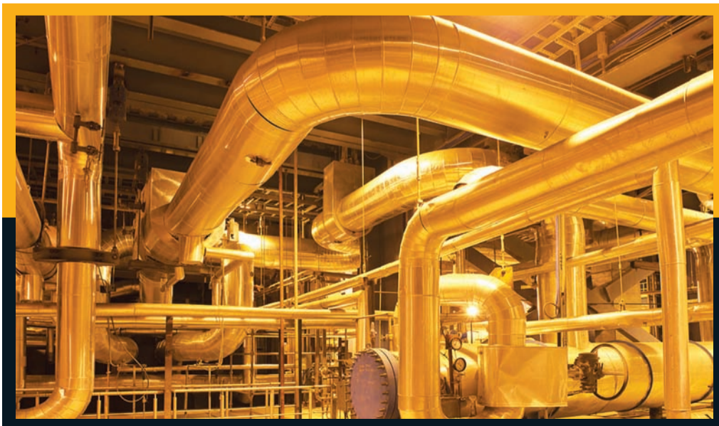
▲ Another view of the Amravati power plant.
